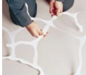
Position; then adhere Pattern Stencil
