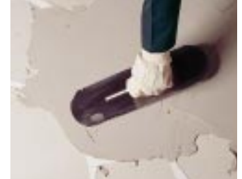
Trowel Finish Coating over Pattern Stencil
