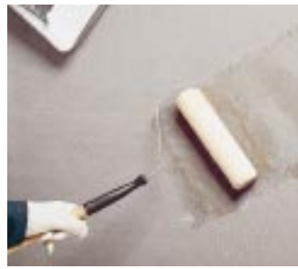
Prep Coat is followed by Grout Coating
