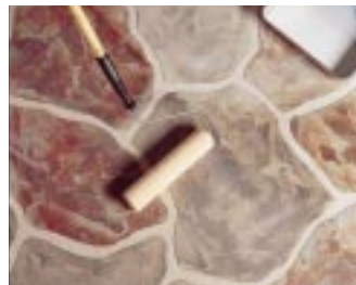
Protect entire surface with Top Coat Sealer
