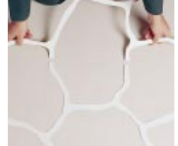
Position; then adhere Pattern Stencil
