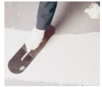
Prep Coat is followed by Grout Coating
